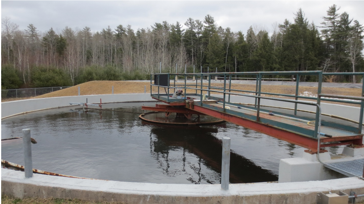
Figure 4.2: Existing Greenwood STP clarifier; surface freezes in winter.
