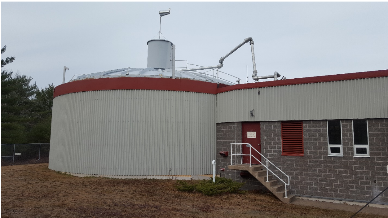
Figure 4.1: Small Anaerobic Digester in Atlantic Canada
