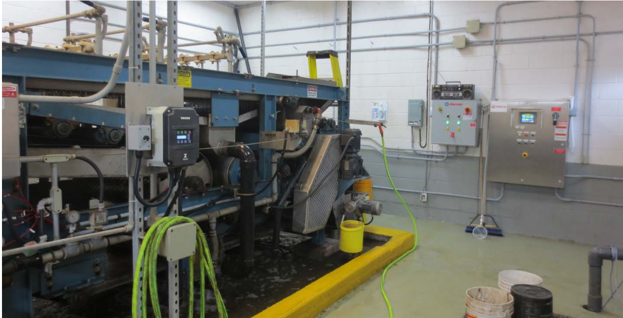
Figure 4.3: Existing Greenwood STP Belt Filter Press
